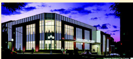
Saratoga Springs City Center
